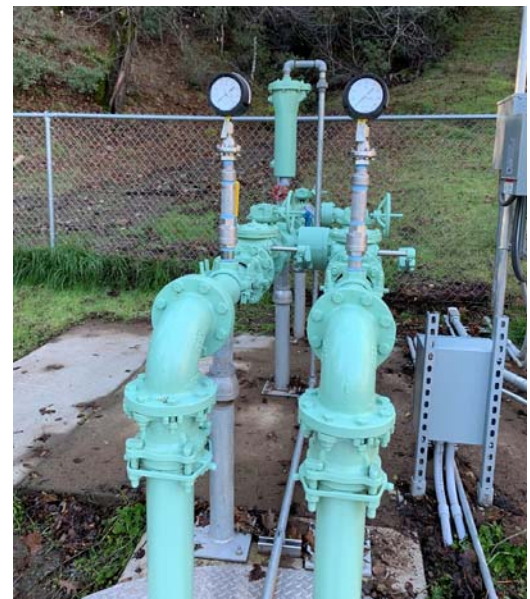
Sewer pump station upgrade
