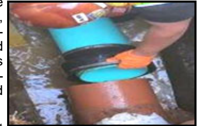
LCSD staff replace sections of broken pipe.
