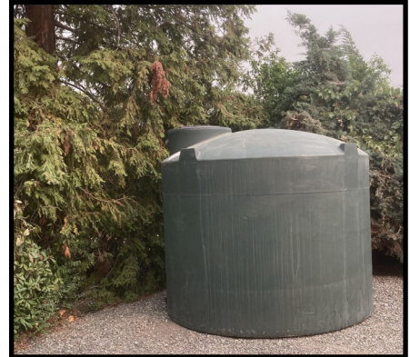
The temporary 2,500 gallon storage tank serving a residence with a dry well.
