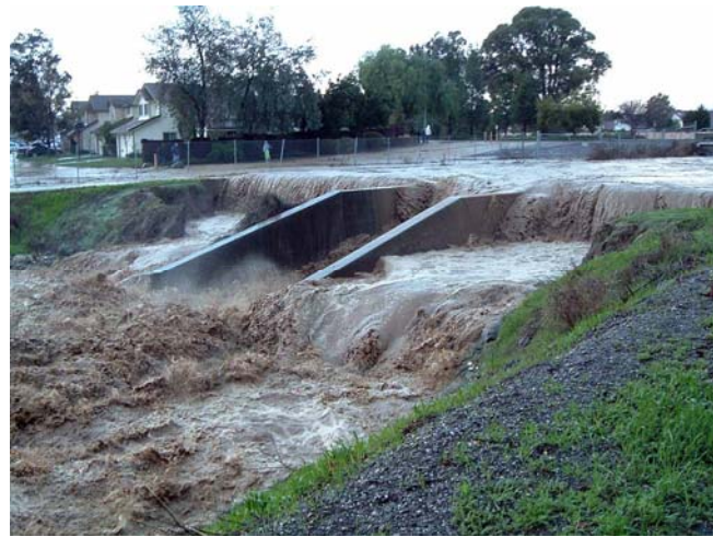
Ulatis Flood Control Channel—Solano County
