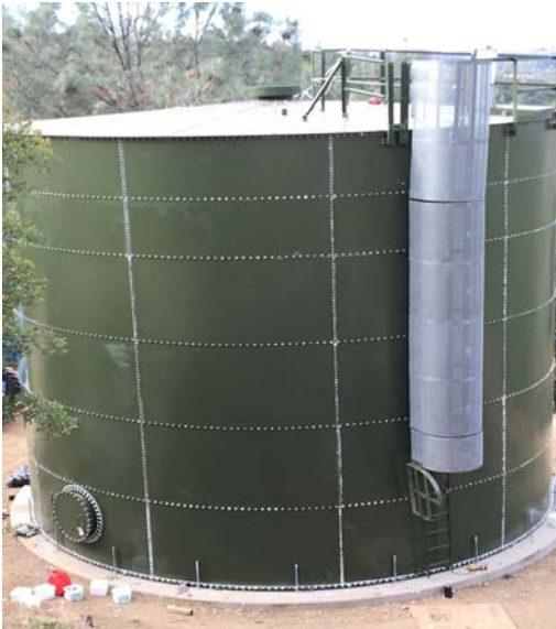
Bolted steel water tank replacement
