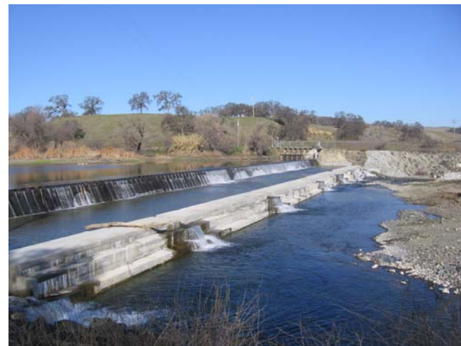
Capay Dam—Yolo County
