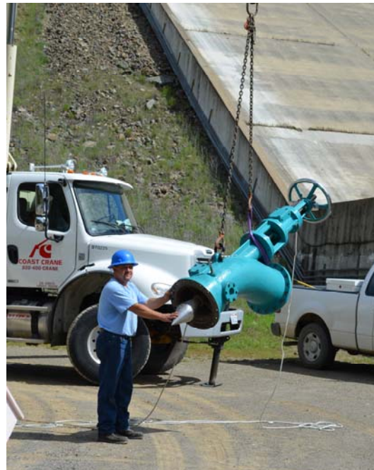
Hydroelectric plant maintenance—Yolo County
