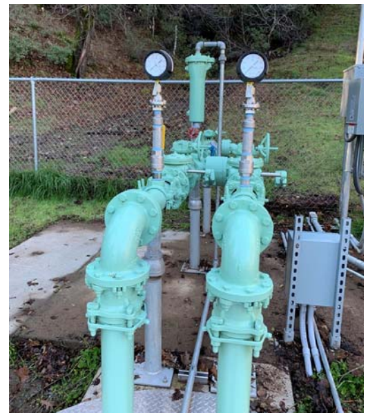
Sewer pump station upgrade
